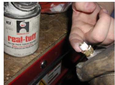
Figure 16 Sealant Used on Plug Threads
