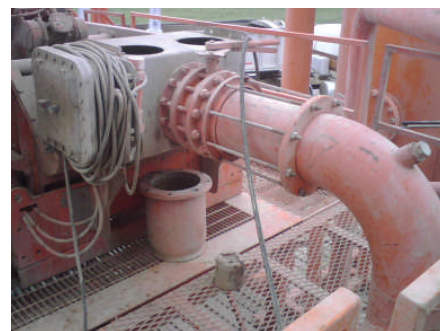
Figure 10 Inlet Pipe & Flange Connected to Header Box
